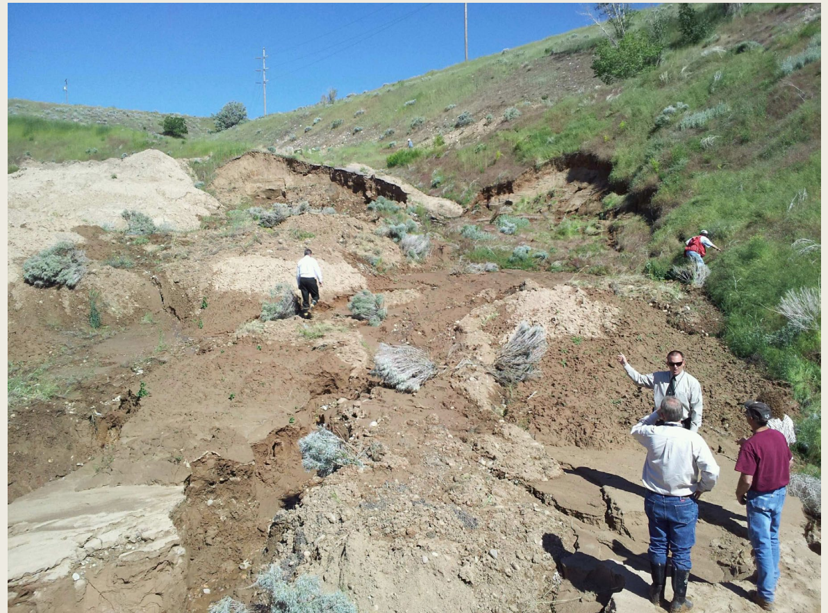
Staker Parson gravel pit north bank seepage and sluffing circa June 8, 2011. Provided by Jones and Associates: Consulting Engineers
