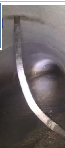
Illicit Connection into Storm Drain
