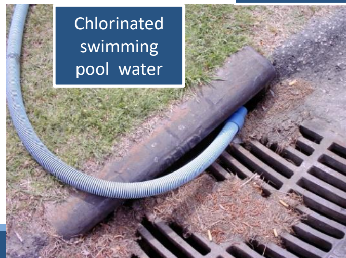
Illicit Connection into Land Drain
