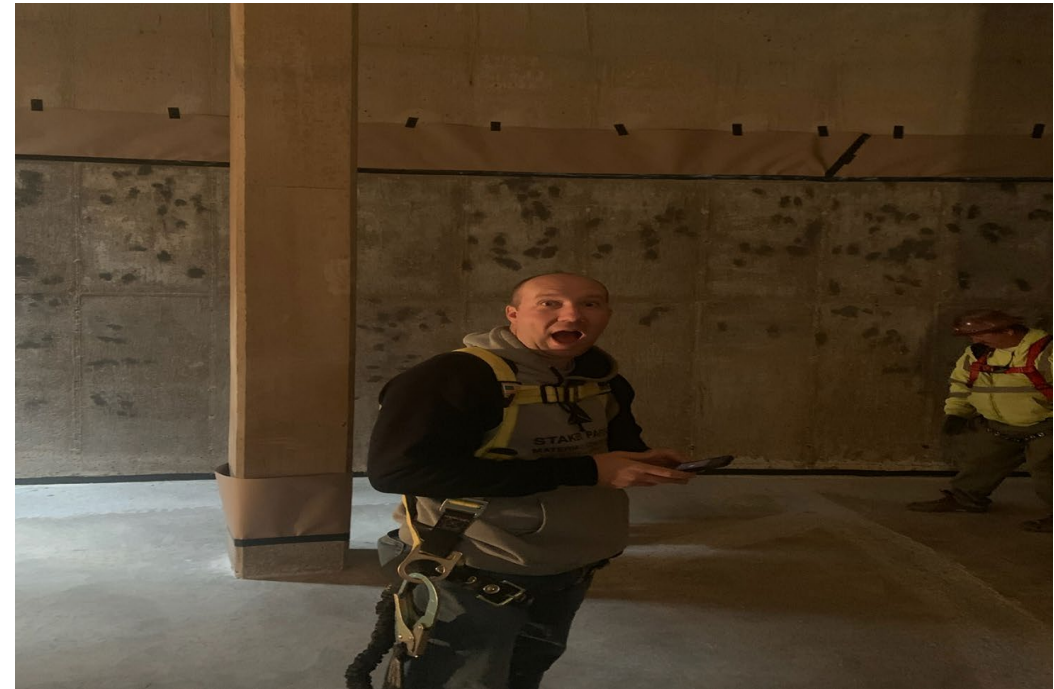
INSIDE REPAIRS ON WEST END TANK
