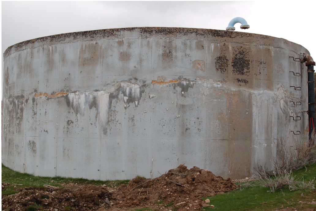
OLD TANK THAT WAS REMOVED
