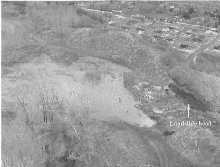
Figure 5. View looking northwest at the pond in the gravel pit and the landslide head (arrow). A berm was placed between the pond and the landslide to prevent water from flowing onto the landslide. Photo taken on the morning of April 10, 2005, by Davis County Sheriff's Office personnel.
