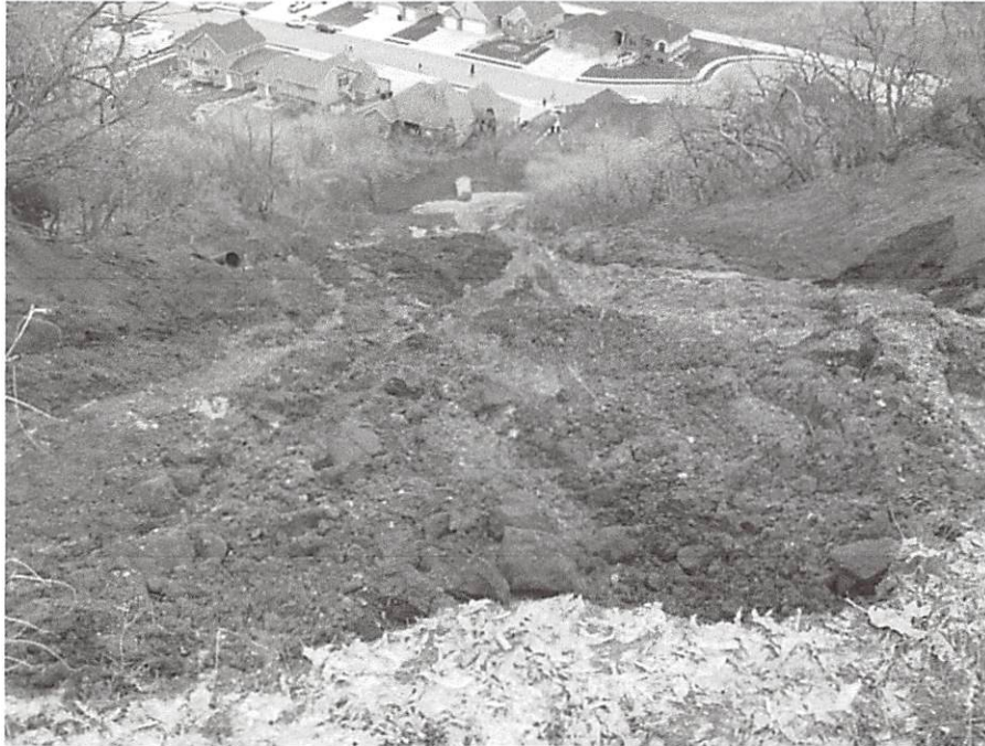
Figure 7. View looking down the landslide flow path at the damaged house at 1650 East 7687 South. The culvert in the lower slide path above the house was originally in the gravel pit. Subsequent water flow eroded the right side of the landslide.
