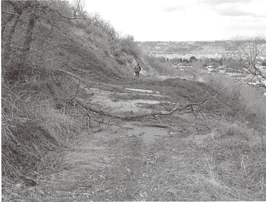
Figure 10. Landslide material deposited on a dirt road midslope above the Davis-Weber Canal.
