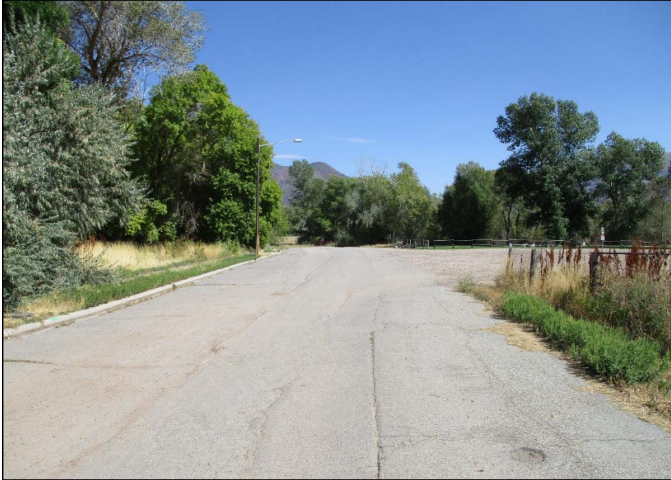
Viewing east along 6650 South Street (subject residential land on the right)
