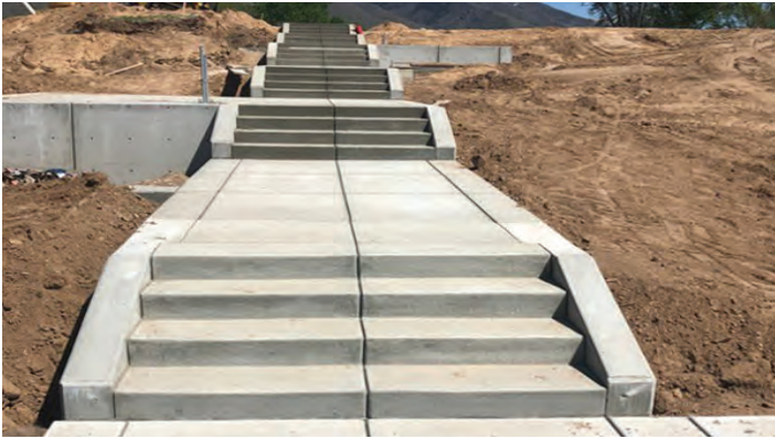
STAIRS & SITE CONCRETE
